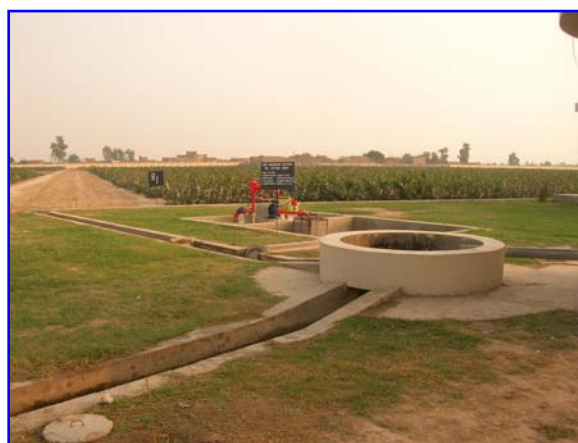
Figure 3. Drip irrigation system installed for cotton at NIAB, Faisalabad using materials imported from China.
