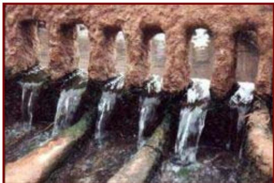
Figure 5. Water "metering" through a distribution weir on a Foggara in Algeria
